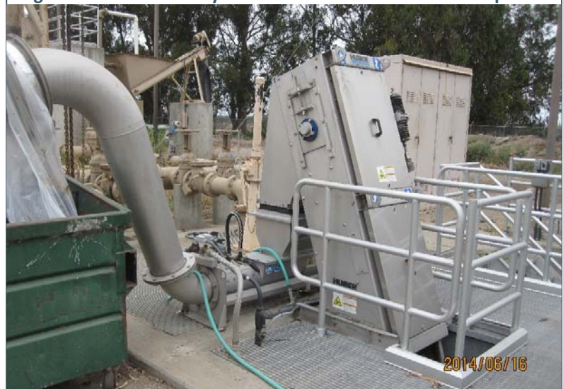
Figure 8-5: Mechanically-cleaned Screen and Washer-compactor
