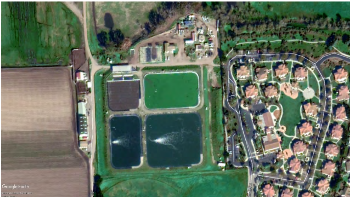
Figure 9-2 Guadalupe Wastewater Treatment Plant
