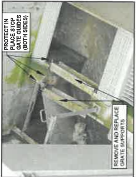
GRATE REPAIR PLAN NOT TO SCALE
