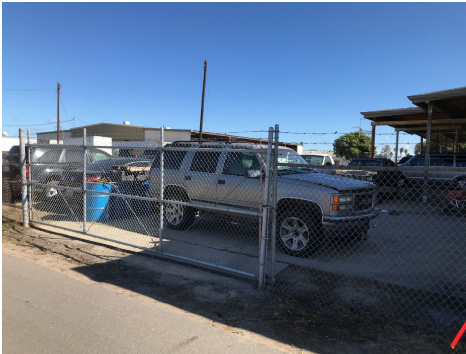
View from west to East (Fence structure is in generally good shape. Vehicles blocking alley access to 333 Guadalupe St at the gate located 200 feet from the Southwest corner of the lot. (Removal of obstructions and Knox padlocks would need to be added)
