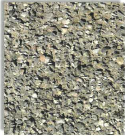
Weathering or Raveling
