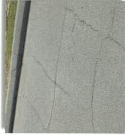
Block Cracking
