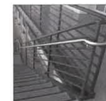
10. METAL GUARD RAILING
