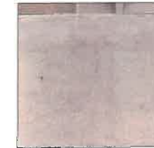
01. EXISTING PLASTER (PINK)
