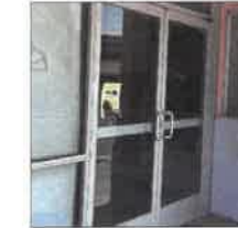
04. EXISTING GLAZING & FRAMING
