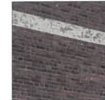
03. EXISTING BRICK & CONCRETE
