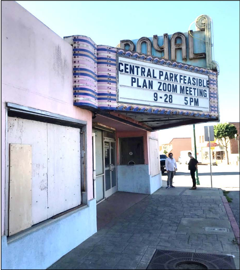
Plate 6. Royal Theater façade, facing south.
