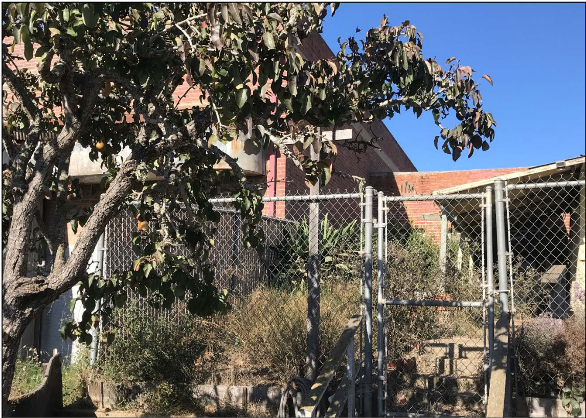
Plate 14. Overview of east and north elevations, facing west.
