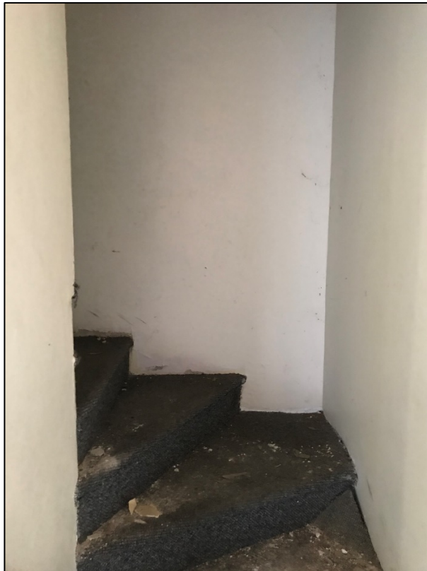
Plate 20. Staircase to second floor projection room.
