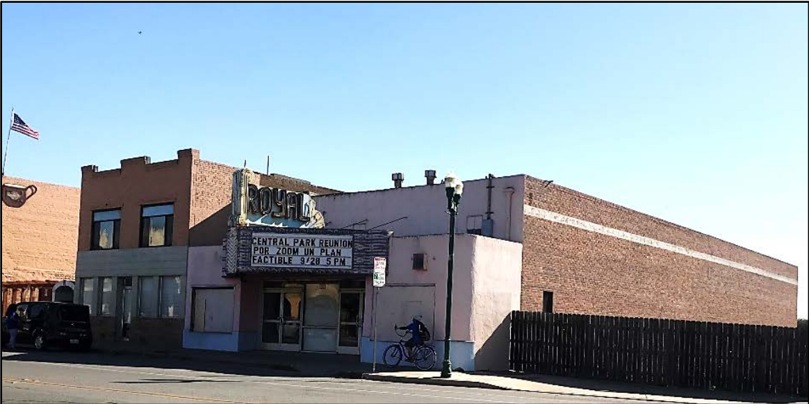
Plate 1. Overview of Royal Theater, facing northeast.
