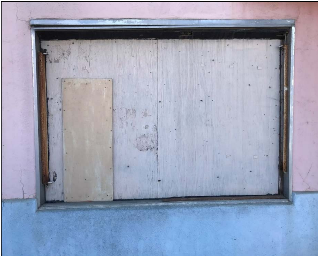
Plate 8. Poster frame on north end of façade.
