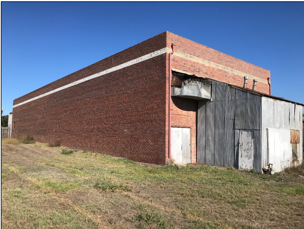
Plate 12. Overview of south and east elevations, facing northwest.
