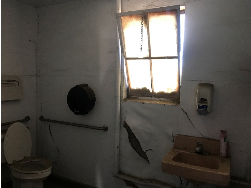
Plate 19. 2/2-light hopper window in ladies room.
