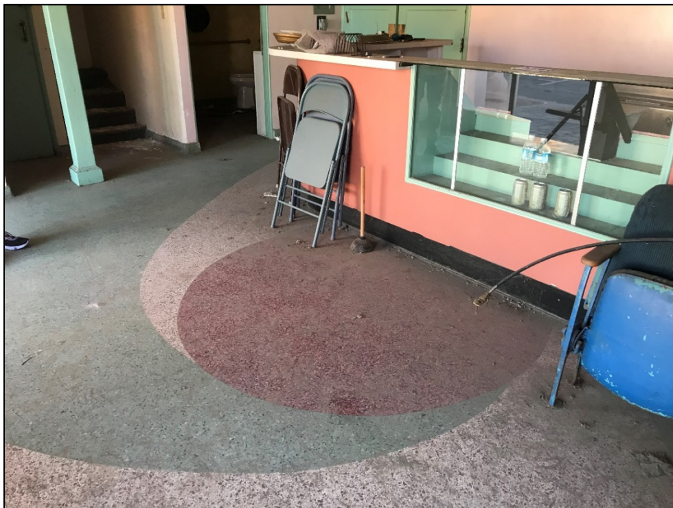
Plate 16. Decorative floor in lobby. Men's restroom and steps to projection room in background.
