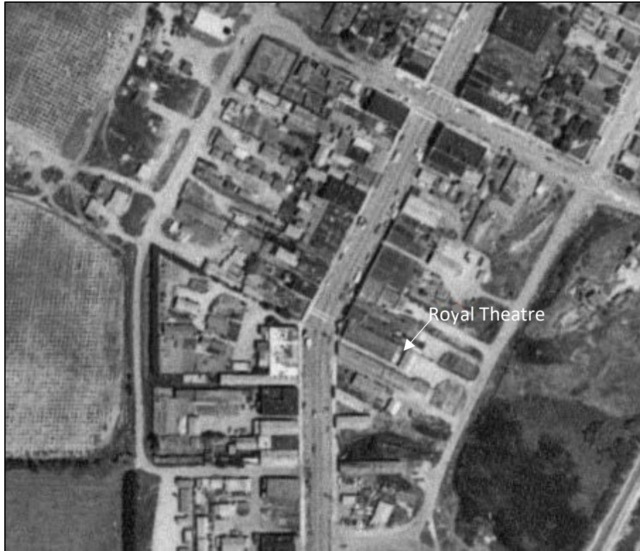
Figure 11. Aerial photograph of Guadalupe, May 4, 1954 (btm-1954_10k-87).
