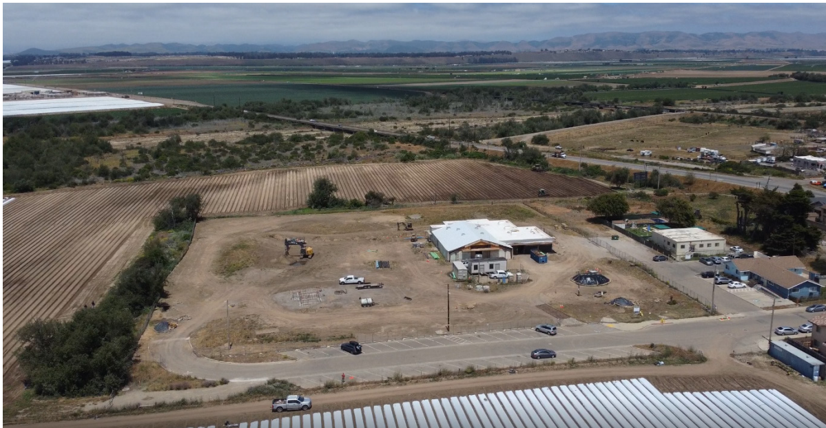
Figure 16: LeRoy Park under reconstruction in May 2021 (Photo Credit: Eric Larson)
