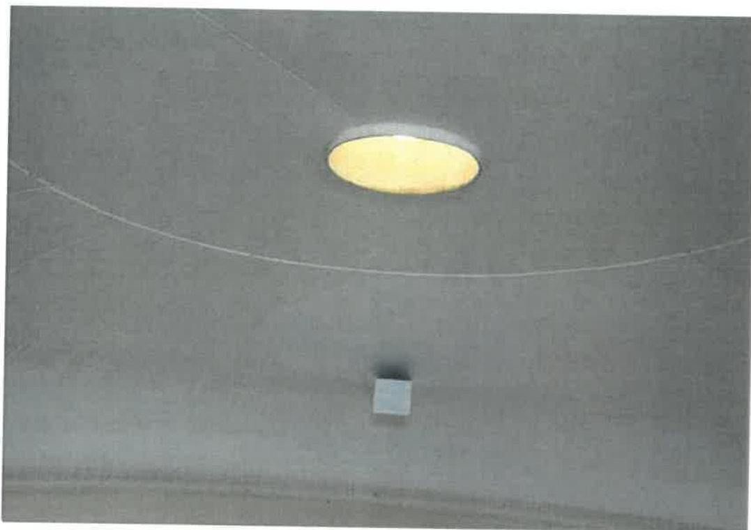
Interior view of the vent and overflow.
