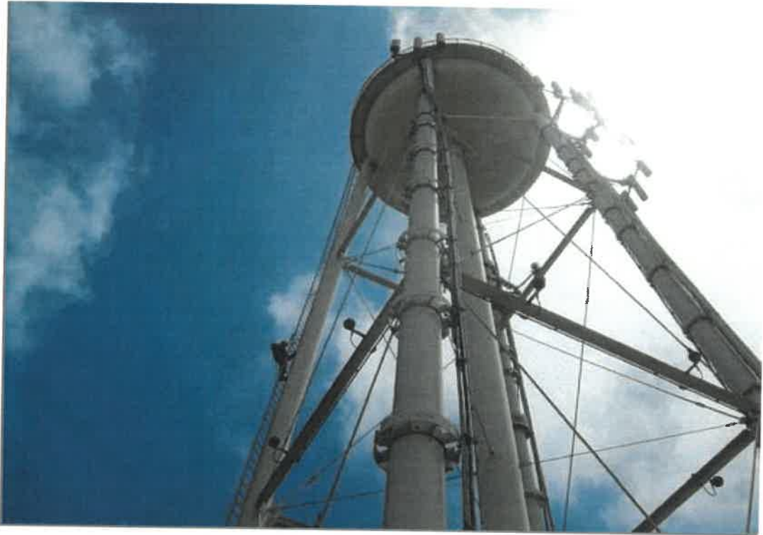
Overall view of the tank.
