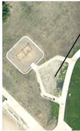
Existing Aerial View
