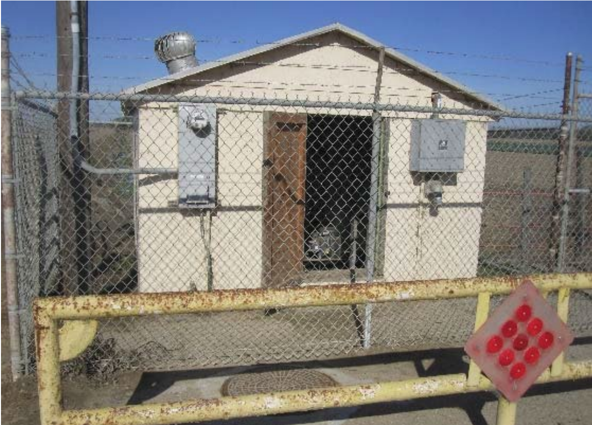
Figure 9-3 Pioneer Street Lift Station
