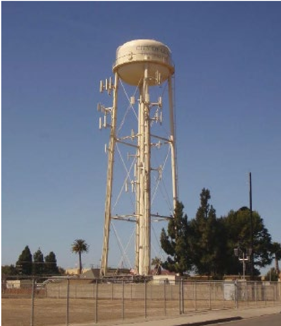
Figure 9-1 Elevated Water Tank at Pacheco and 10 th Street
