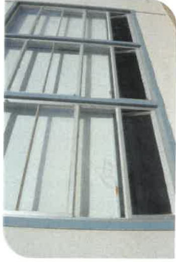
Windows from another era
