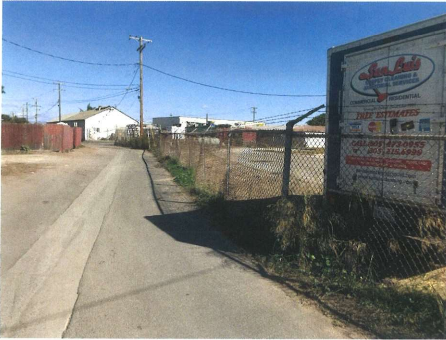
View from South to North (Fence structure is in generally good shape. Repair of fence bindings, straightening of fence poles, tightening of the fence, and weed abatement required.)
