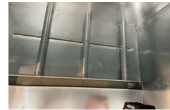
Steel Plated Walls
