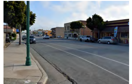
Figure 3.3.6 Existing street condition
