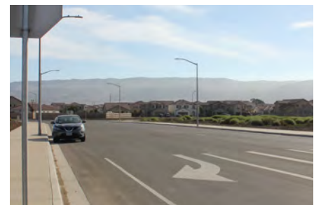
Figure 3.3.4 Street existing condition
