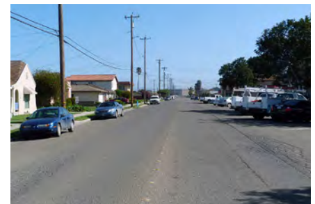
Figure 3.3.5 Street existing condition
