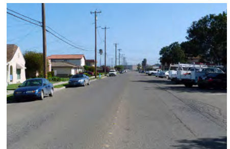
Figure 3.3.5 Street existing condition
