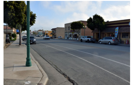
Figure 3.3.6 Existing street condition
