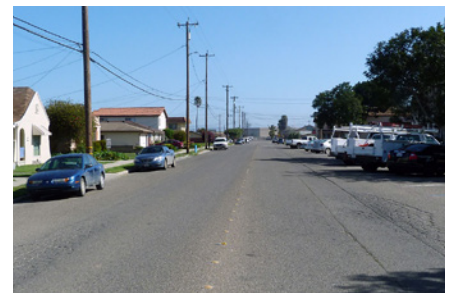
Figure 3.3.5 Street existing condition
