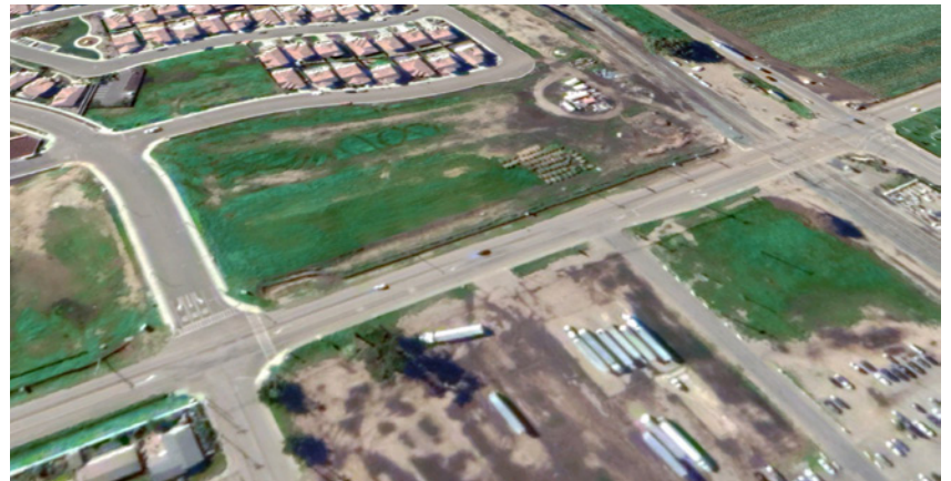
Figure 3.4.12 (Top) Conceptual rendering of potential improvements to West Main Street and Pasadera, including commercial development oriented to the street, enhanced connections to and from the neighborhood, and a roundabout at the intersection of West Main Street and Obispo Street
