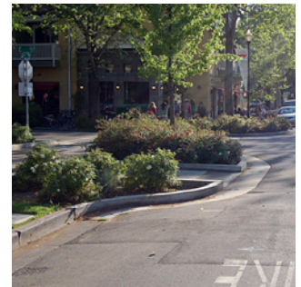
Figure 3.2.3. Curb extension at an intersection.
