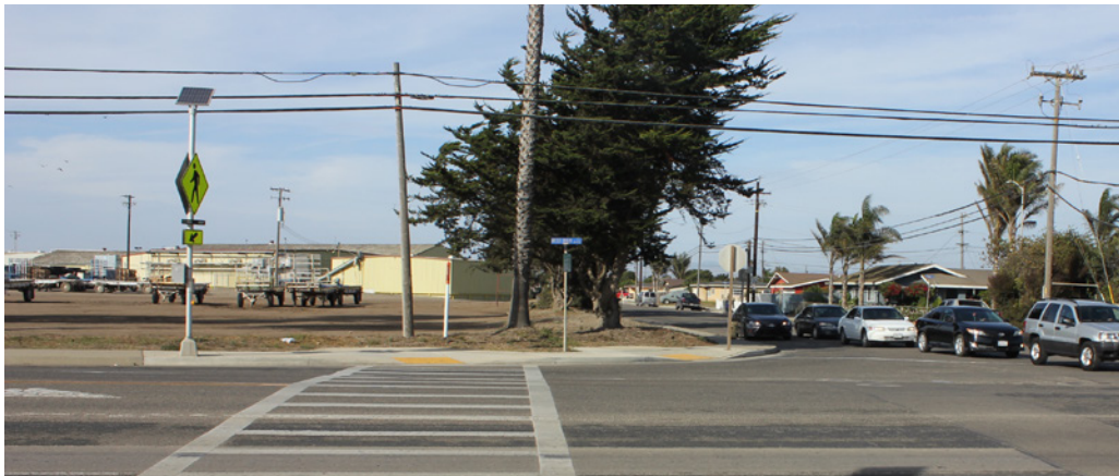
Figure 3.2.8 High-visibility crosswalk markings and Rectangular Rapid Flashing Beacons on West Main Street
