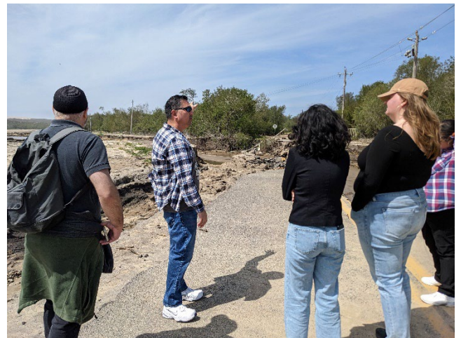
Viewing the flood damage to West Main Street near the dunes during the community tour (Credit: Megan McConville)
