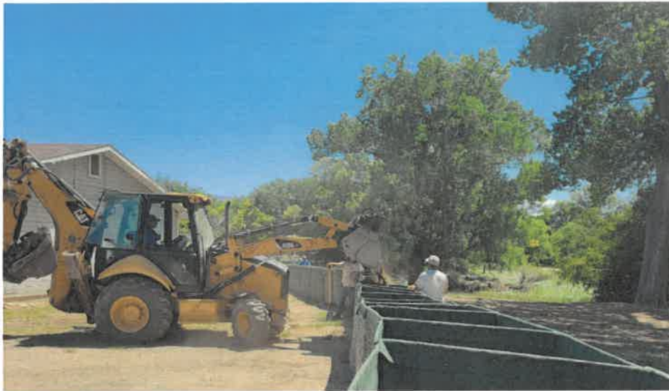
Figure 2. HESCO Baskets Being Filled
