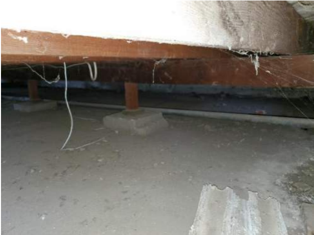
Figure 41: Post, Beam, and Pad Foundations at Raised Floor.
