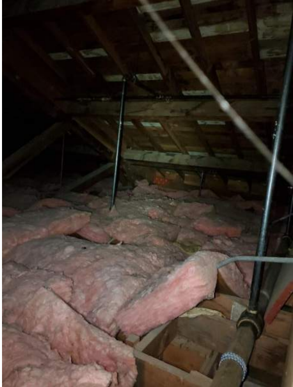
Figure 13: Interior Roof Framing at Gymnasium 07
