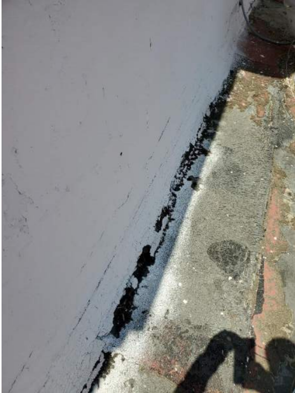
Figure 46: Roof at Mechanical Equipment.
