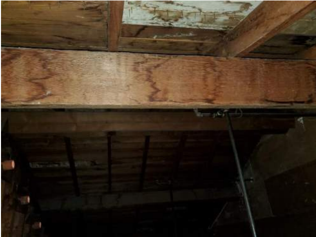
Figure 9: Interior Roof Framing at Gymnasium 03
