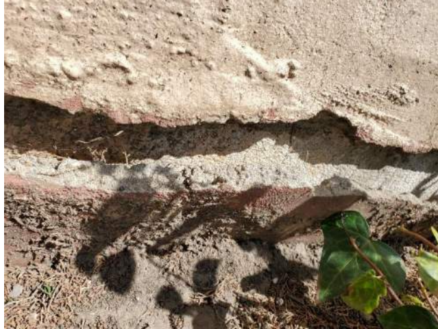
Figure 56: Exterior Grading and Stucco at Foundation 03.
