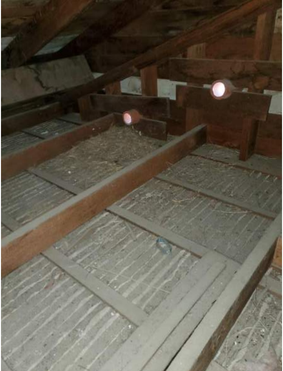
Figure 14: Interior Roof Framing over Main Entry, Gymnasium 08
