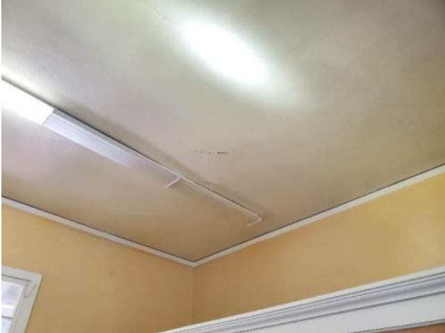
Figure 23: Interior Ceiling Finish.
