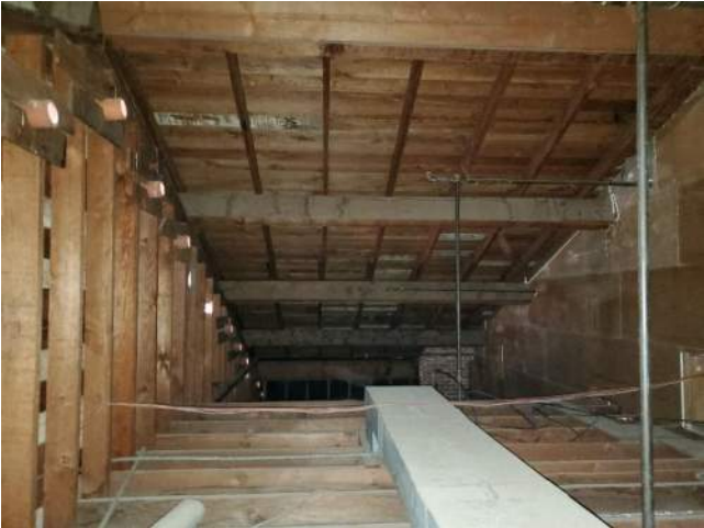
Figure 8: Interior Roof Framing at Gymnasium 02
