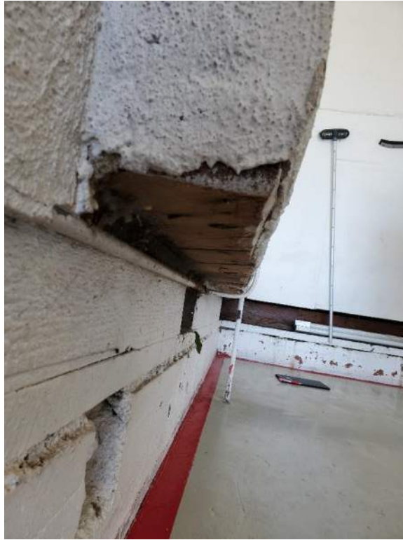
Figure 21: Cantilevered Sheathing at Raised Floor.
