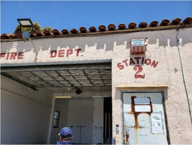
Figure 19: Exterior Wall at Fire Department 01.
