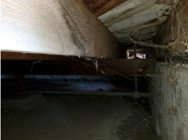
Figure 40: Crawl Space Framing and Sheathing.
