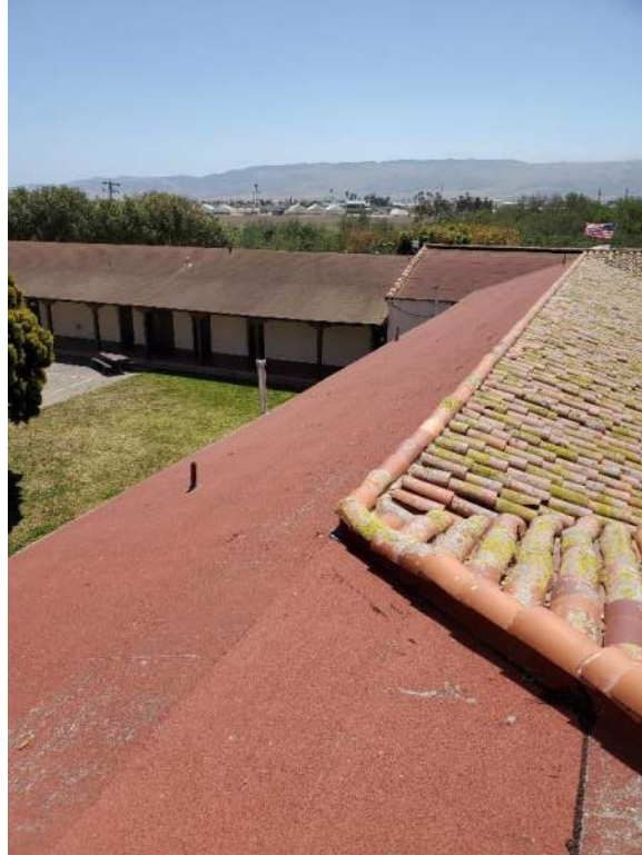
Figure 43: Roof Composition at Courtyard 01.
