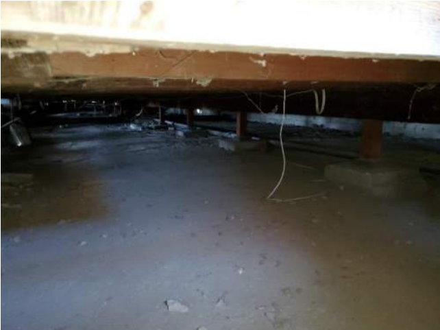
Figure 42: Interior Support Line at Raised Floor.
