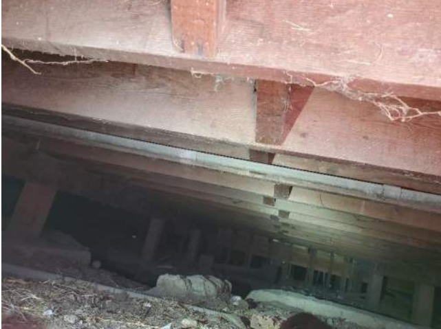
Figure 18: Crawl Space Below Gymnasium.
