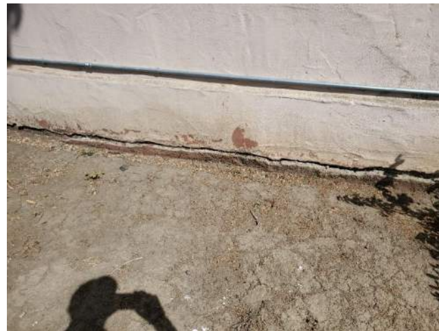
Figure 55: Exterior Grading and Stucco at Foundation 01.
