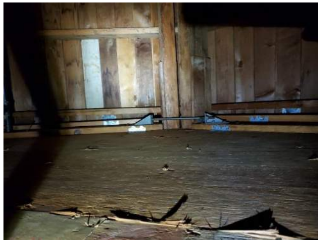
Figure 12: Interior Roof Framing at Gymnasium 06
