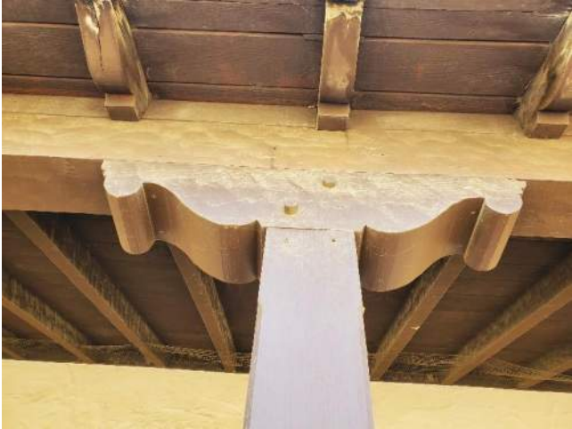
Figure 31: Beam to Column Connection at Colonnade.
