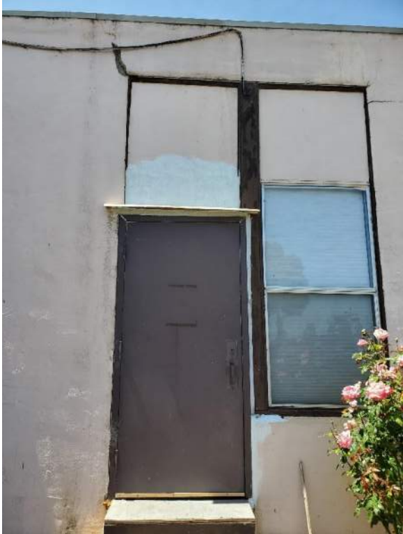
Figure 35: Exterior Wall and Infill at Courtyard.
