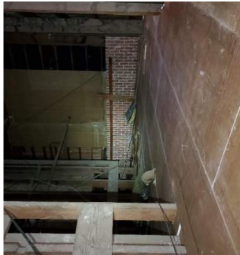
Figure 11: Interior Roof Framing over Main Entry, Gymnasium 05
