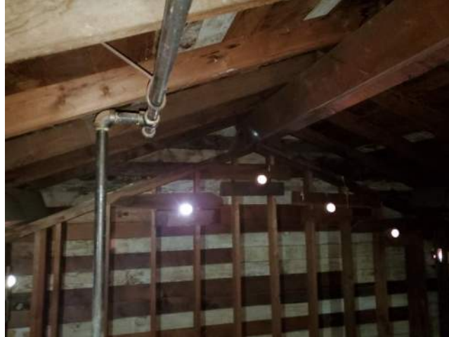
Figure 10: Interior Roof Framing over Main Entry, Gymnasium 04
