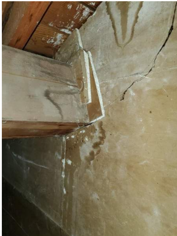
Figure 22: Beam to Support
