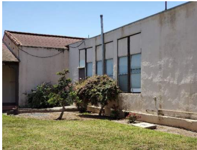
Figure 33: Exterior Wall at Courtyard 02.
