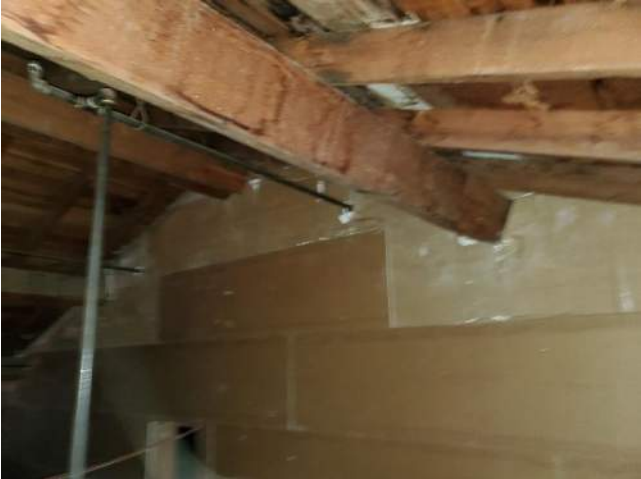
Figure 7: Interior Roof Framing at Gymnasium 01
