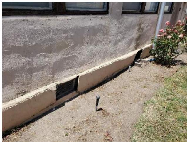
Figure 34: Exterior Crawl Space Vents at Courtyard.
