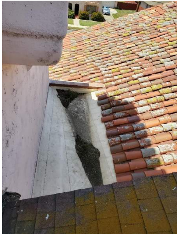
Figure 47: Sloping and Drainage at Roof.
