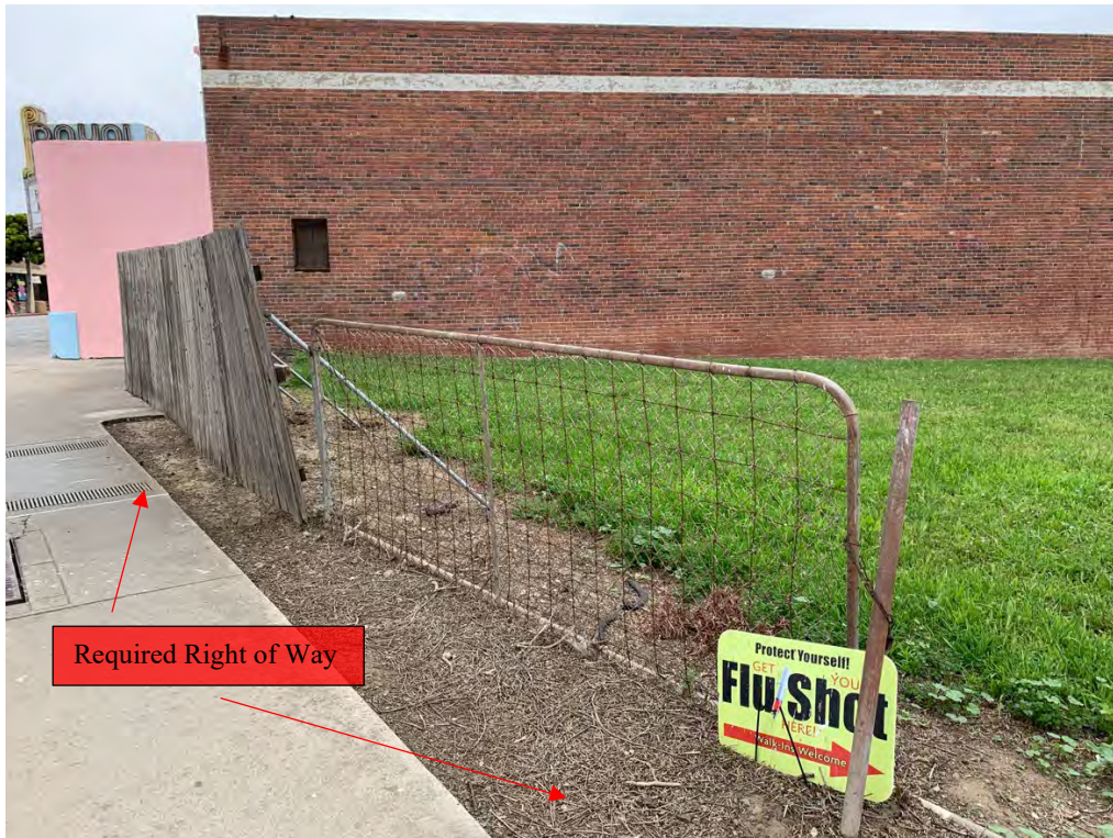
Required RW with wooden fence and gate facing north (Photo by M. Linder 4/22/2024)
