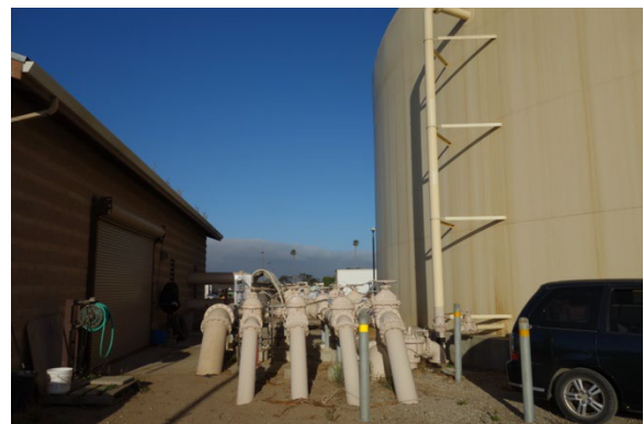
(#12) Exterior Inlet, Overflow, and Drain
