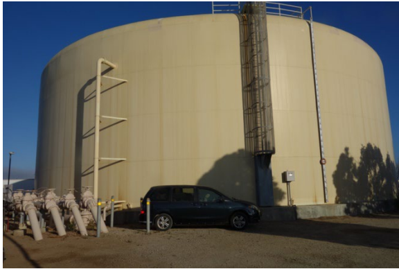
(#13) Site, Exterior Ladder, Inlet, and Overflow
