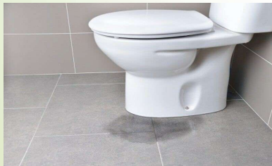
Fix Leaking Toilet Immediately
