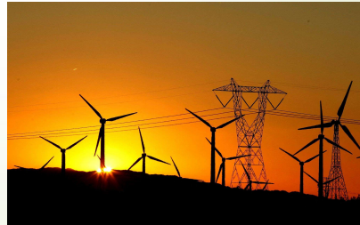
Upgrading the power grid
